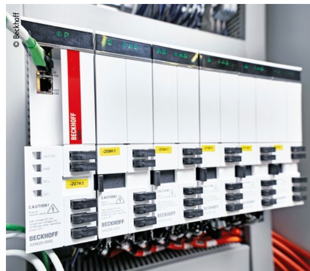
The compact AX8000 multi-axis servo system and OCT connection technology save valuable space in the control cabinet.
