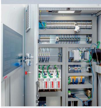
The view inside the control cabinet shows the Beckhoff C6030 ultra-compact Industrial PC and the inline connected EtherCAT Terminals (center right) as well as the AX5000 Servo Drives (center) and the 12-inch CP2912 multi-touch Control Panel (left).
