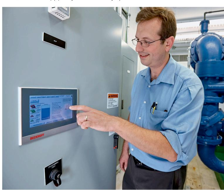
The pumping station is controlled via a CX2020 Embedded PC with directly connected EtherCAT I/Os.
