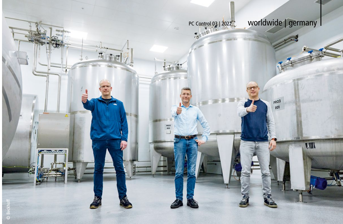
“With Beckhoff, everything just works – you have technology, flexibility, professionalism and the human factor,” sums up Rüdiger John (center), Head of Engineering at Engelhard Arzneimittel, shown with Stefan Maßmann (left) and Andreas Wieners (right), both from Beckhoff Systems Engineering.
