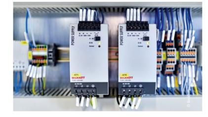
The PS3031-2420-0001 power supplies - 3-phase, 24 V DC devices with 20 A output current and 480 W output power - reliably supply the control technology and, with high efficiency and low heat loss, have a positive effect on system availability
