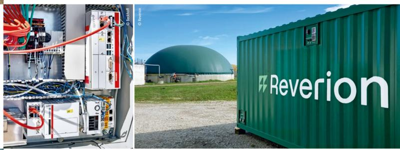
The control architecture uses two computers: a CX2043 Embedded PC (bottom) and a C6930 control cabinet Industrial PC (top, to be replaced in the future by a C6030 ultra-compact Industrial PC).
