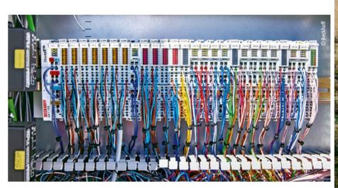
One of numerous EtherCAT Terminal segments in one of the nine control cabinets for control technology and power supply
