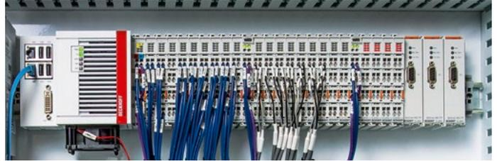
Compact EtherCAT Terminals and CX5140 Embedded PCs from Beckhoff helped iZ Systems reduce its control cabinet sizes by two-thirds in most cases.
