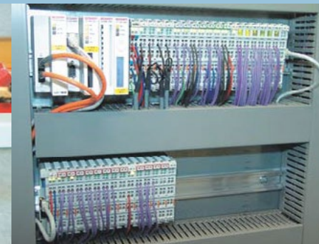
Control cabinet of the gearbox test rig for the tail rotor with the CX1000 Embedded PC
