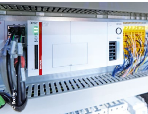
The CX2072 Embedded PC with directly connected EtherCAT and TwinSAFE terminals controls all motion and test sequences.
