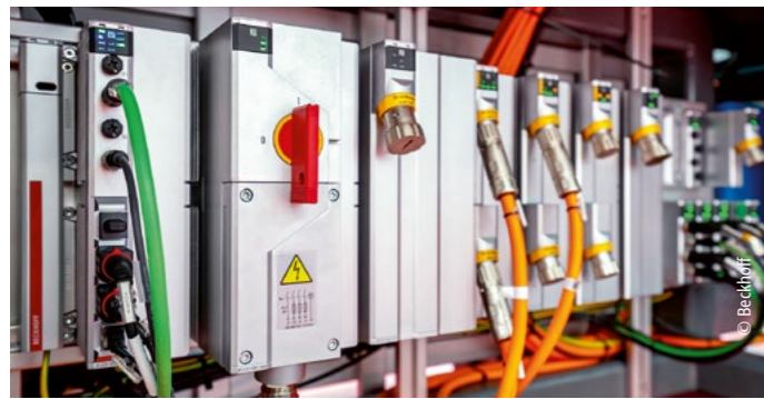
By placing the MX-System in the substructure of the winding machine, the classic control cabinet can be dispensed with completely.
