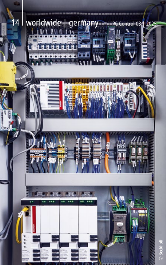
Control cabinet of the mySaw ring sawing machine with the CX5240 Embedded PC and the connected EtherCAT and TwinSAFE Terminals (top) and the AX8000 multi-axis servo system (bottom)
