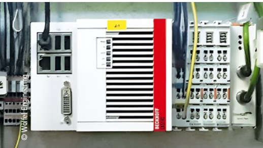
The CX5140 Embedded PC – with directly attached EtherCAT Terminals and EP3752-0000 I/O box modules connected via EtherCAT – reliably collects all the data required for condition monitoring.
